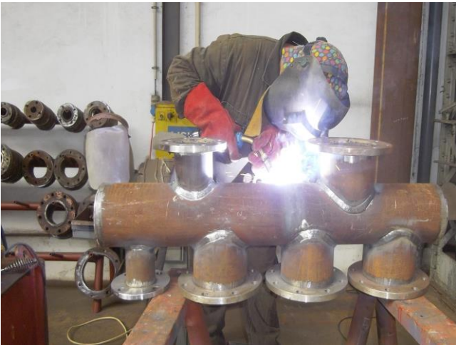
Welding of pipes in workshop
