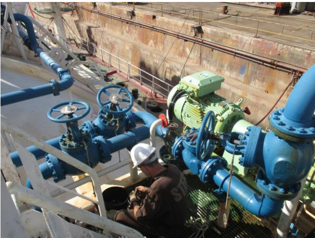
Removal cargo line valves
