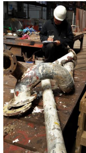
Pipe fabrication in our workshop
