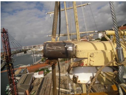
Mast repair at about 60 m height
