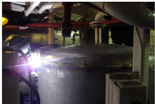
Boiler repair
