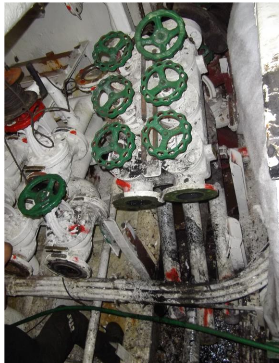
Removal pipes and valves in ER
