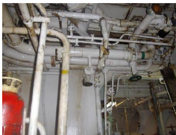
View of status of pipe in ER
