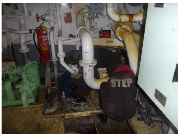
Removal of seawater pipes
