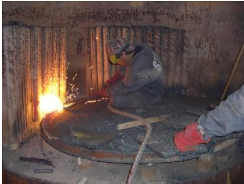
Removal of damaged areas
