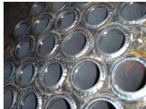
Welded tubes using GTAW and SMAW
