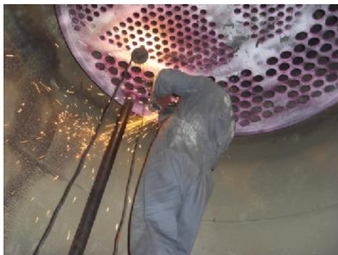
Cleaning and grinding Top Tube Plate
