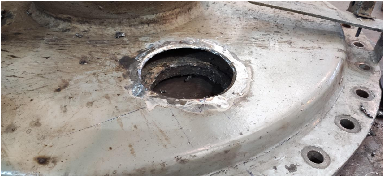
Preparation of the new pipe branch and other parts.
