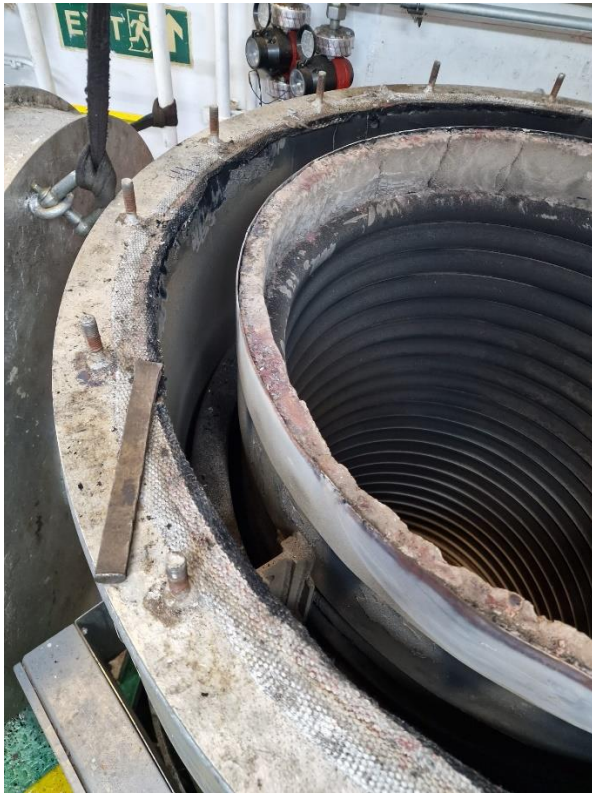
1. General view of the boiler, bottom and upper refractory areas, found damaged
