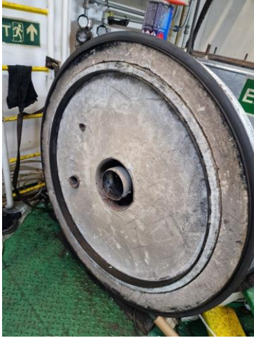
3. Boiler Cover repaired with new steel ring in the seal box.
