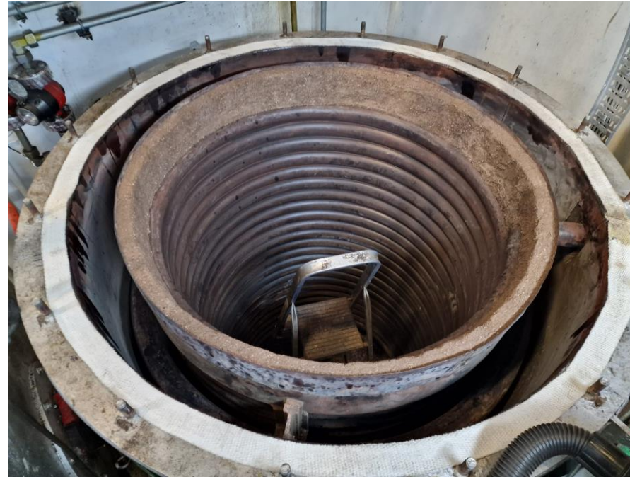
5. Refractory repaired. New seal applied on flange.
