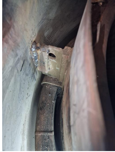
4. Internals already repaired by welding
