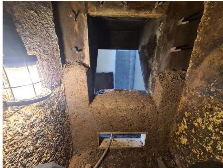
New refractory castable application
